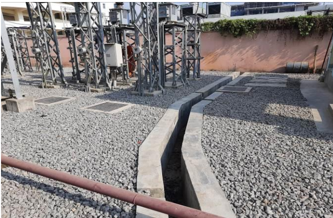
Drainage within the 132/33 kV GMCH (New) S/S
