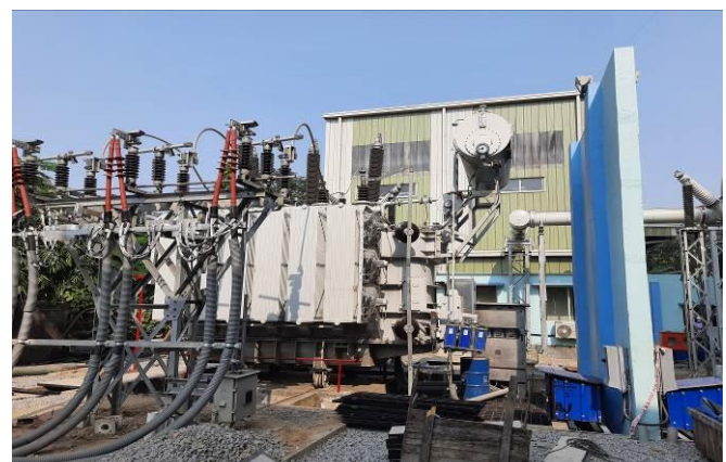
Fire Wall and EPFES at 132/33 kV Paltanbazar GIS S/S
