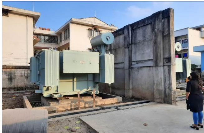
Fire Wall at 33/11 kV GMCH and Arya College S/S
