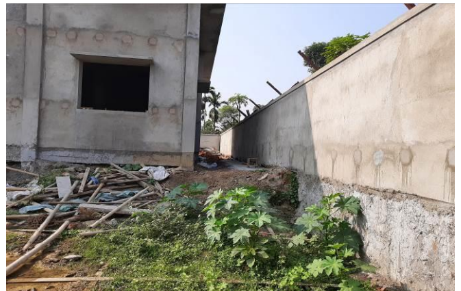
Under Construction Drainage within the 33/11 kV Tarun Nagar (New) S/S
