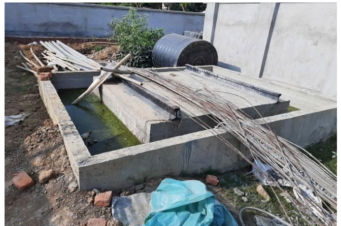
Oil Spill Containment Systems at 33/11 kV Arya College and Tarun Nagar S/S
