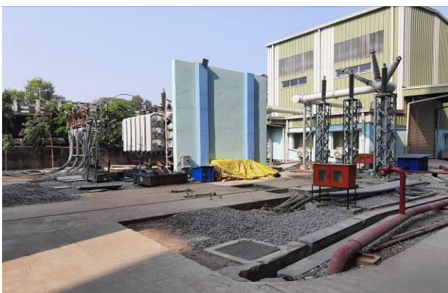
Fire Wall and EPFES at 132/33 kV Paltanbazar GIS S/S
