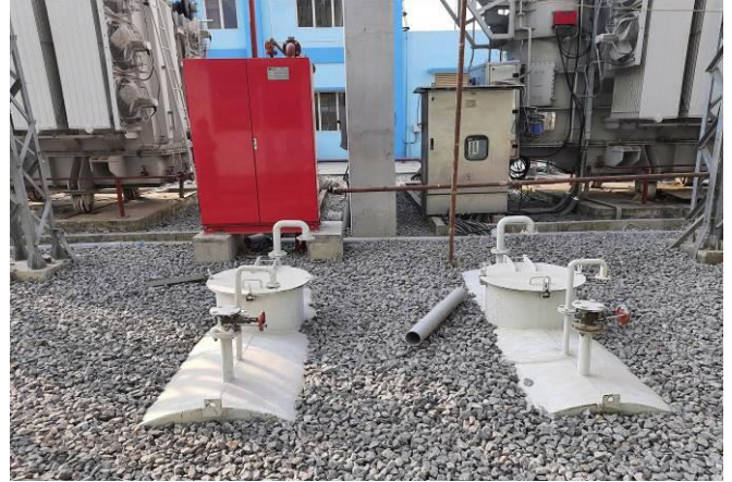
Oil Spill Containment Systems 132/33 kV and 33/11 kV GMCH (new) S/S
