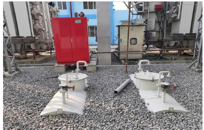
Fire Wall and EPFES at 132/33 kV GMCH GIS S/S
