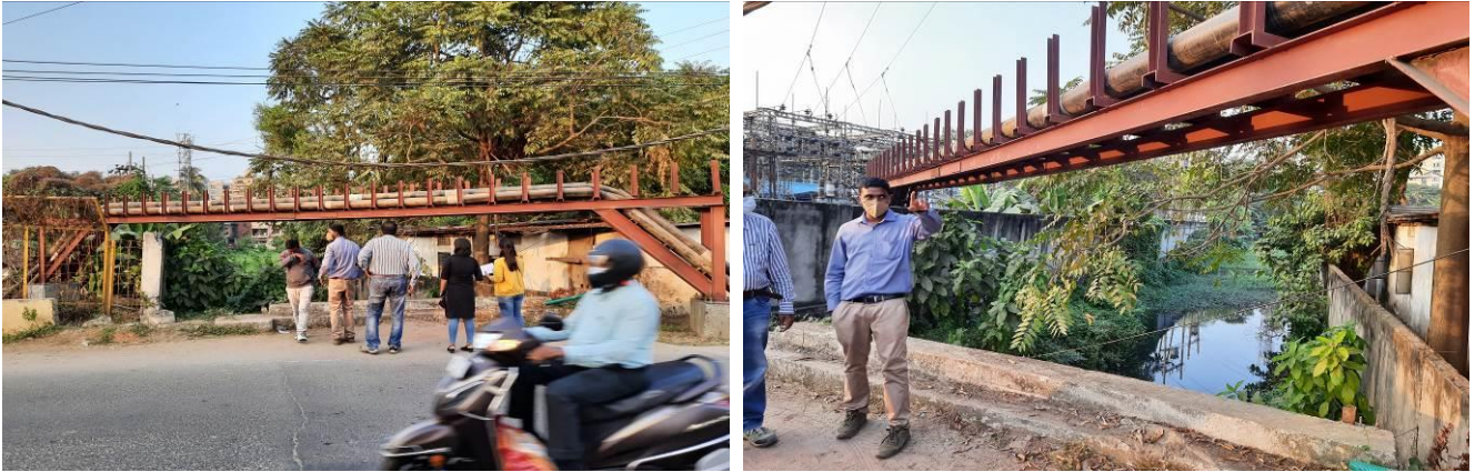
Arrangement to Avoid Interference with Drainage in GMCH – Ulubari 33 kV UG Cable
