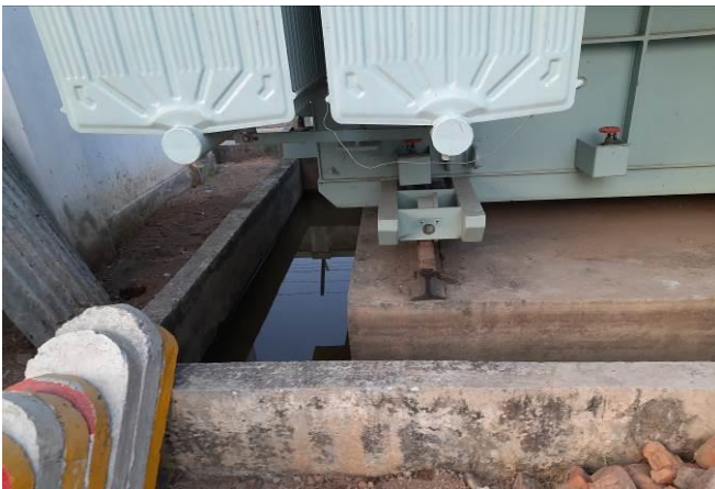
Oil Spill Containment and Sewerage Systems at 33/11 kV GS Road S/S
