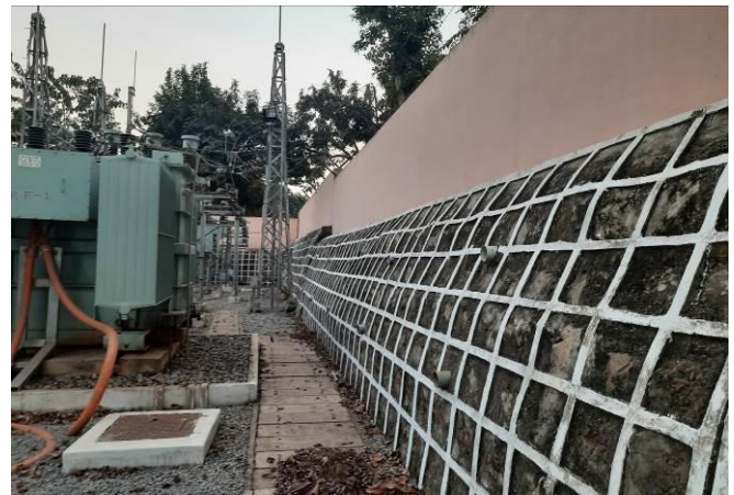
RRM Wall at 33/11 kV Chabipool Substation
