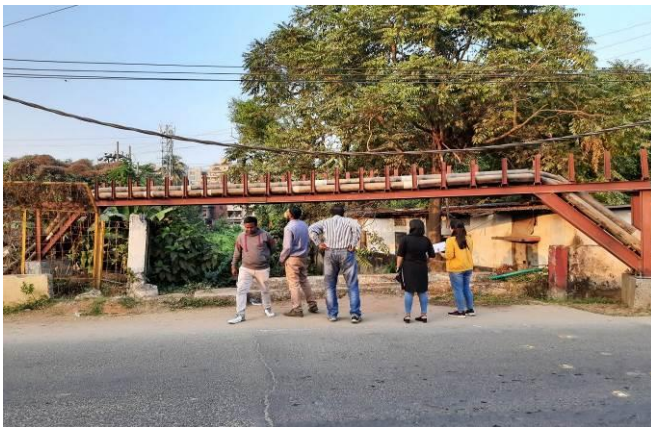
Overhead Section of GMCH to Ulubari Line to Cross Nala
