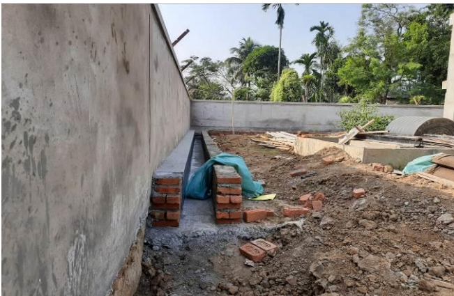
Under Construction Drainage within the 33/11 kV Tarun Nagar (New) S/S
