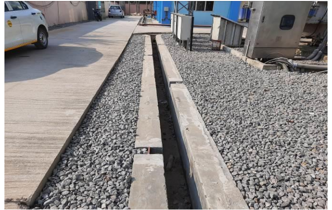
Drainage within the 33/11 kV GMCH (New) S/S
