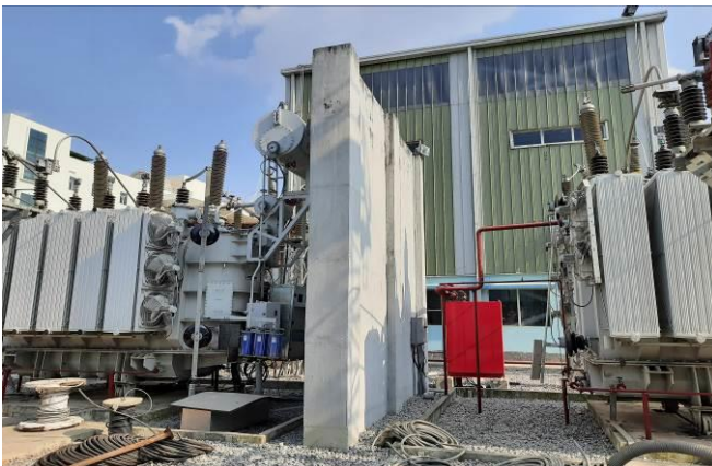
Fire Wall and EPFES at 132/33 kV GMCH GIS S/S
