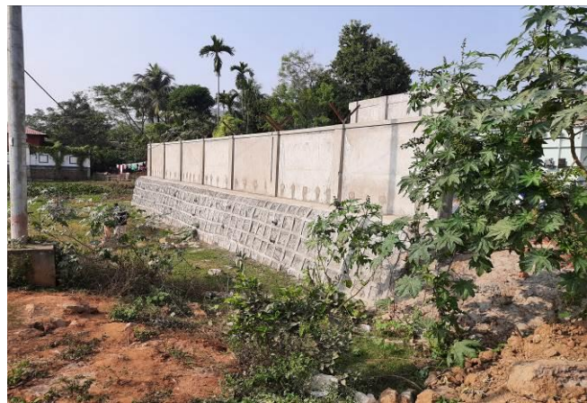
RRM Wall at 33/11 kV Tarun Nagar Substation
