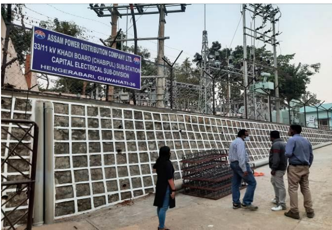
RRM Wall at 33/11 kV Chabipool Substation
