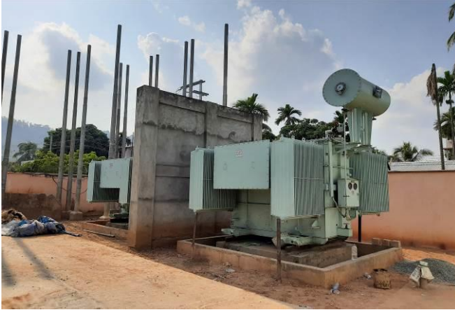
Oil Spill Containment Systems 132/33 kV and 33/11 kV GMCH (new) S/S
