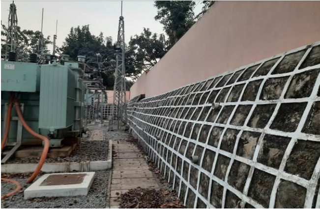
Oil Spill Containment and Sewerage Systems at 33/11 kV Chabipool S/S
