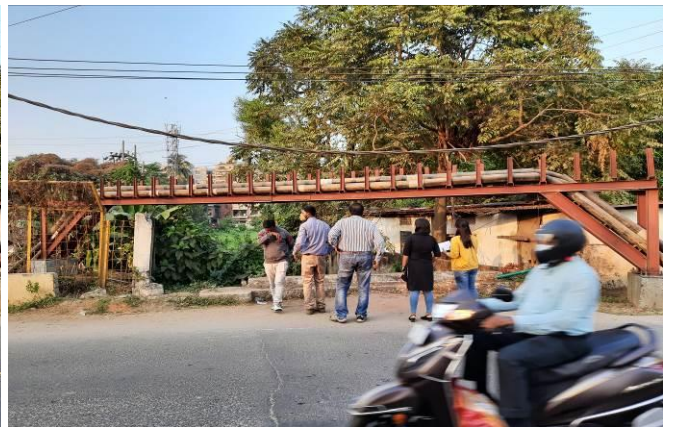
Overhead Section of GMCH to Ulubari Line to Cross Nala
