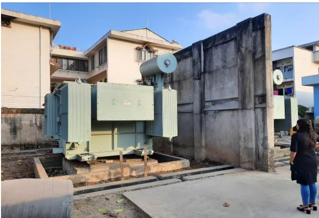
Oil Spill Containment Systems at 33/11 kV Arya College and Tarun Nagar S/S
