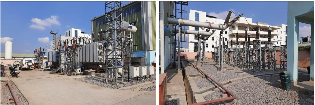
Levelled Surface at 132/ 33 kV GMCH GIS S/S
