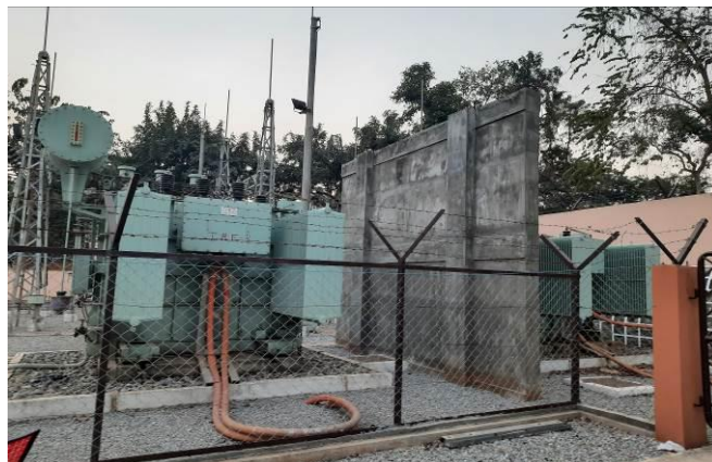
Fire Wall at 33/11 kV GS Road and Chabipool S/S
