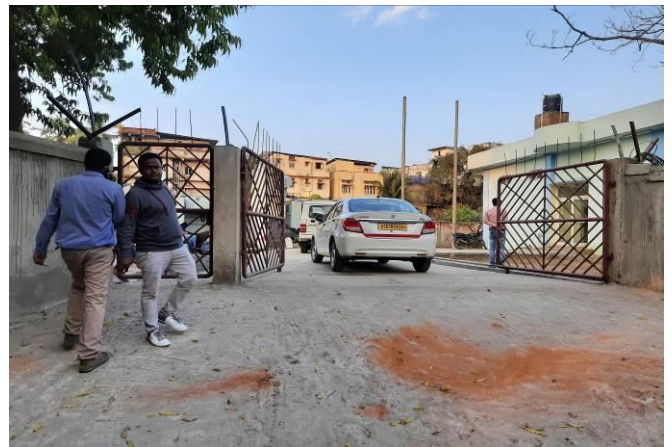
33/11 kV GS Road Substation (New)
