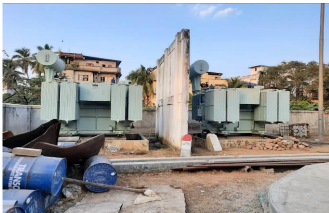
Fire Wall at 33/11 kV GS Road and Chabipool S/S
